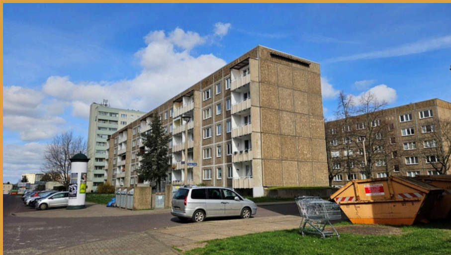
Figure 2: Houses can talk. Older Plattenbau estate, partly Social Housing, Magdeburg Neue Neustadt, 2024
